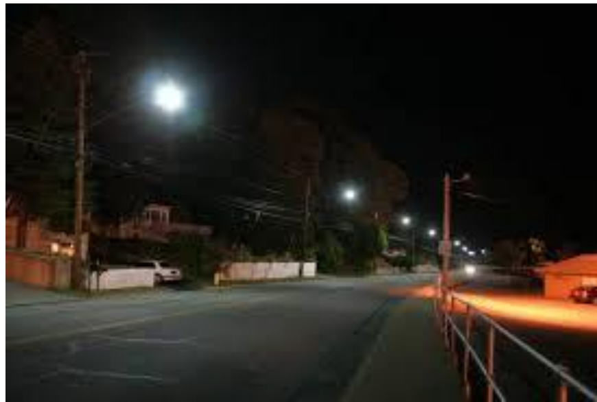
Figure 2: Properly lit roadway [3]
